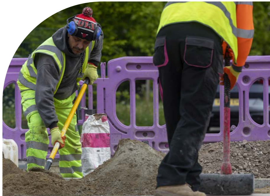
New paving in Northolt
